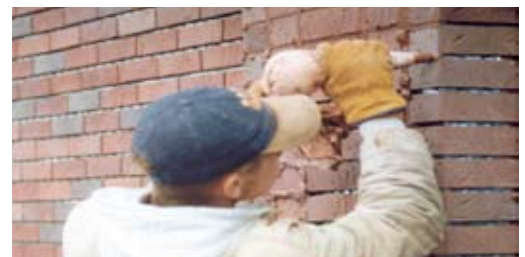
fixing the brick slips
