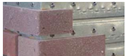
installing corners and returns
