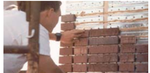
applying the adhesive
